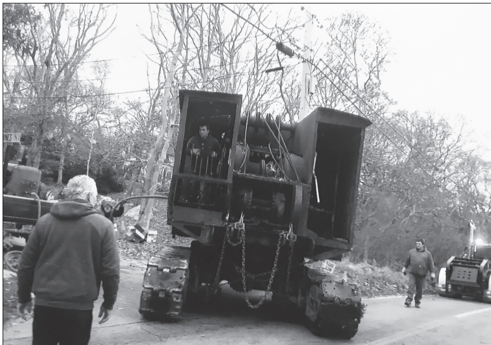
Kevin Stuart, from the Antique Gas Engine Association museum in Schoharie, NY, drives the crane under compressed air power onto Sippewissett Road. The boom and boiler had been transported earlier. November 19, 2018.
